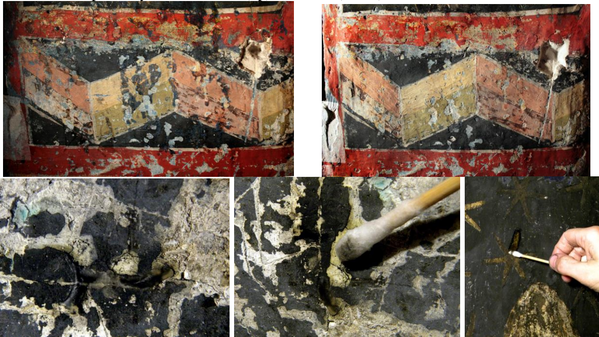
Figure 34. Wax deposits on unstable paint layer
