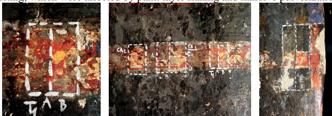
Figure 26. Solubility test on the superficial deposits – AA 10%
