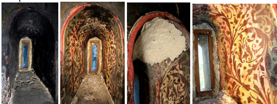
Figures 40 – 43. The small window in the north wall of the Prothesis: the initial state of preservation (left) and the successive stages of removal of hardened deposits from the surface of the paint layer
